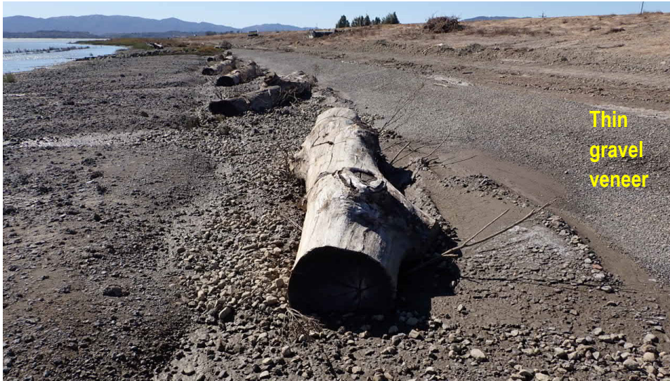
Photograph 13. Gravel veneer thin layer above logs placed before gravel toe berm
