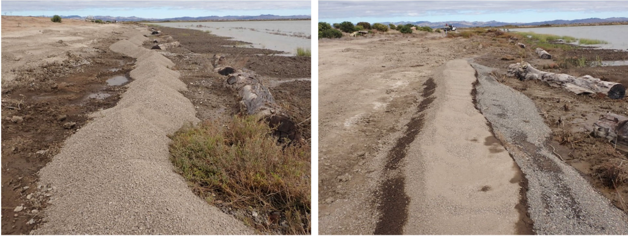
Photograph 12. Sacrificial Berm at Placement and During Wave Reworking
