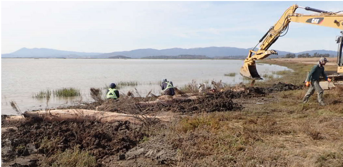
Photograph 11. Installation of logs and fringing coyote brush
