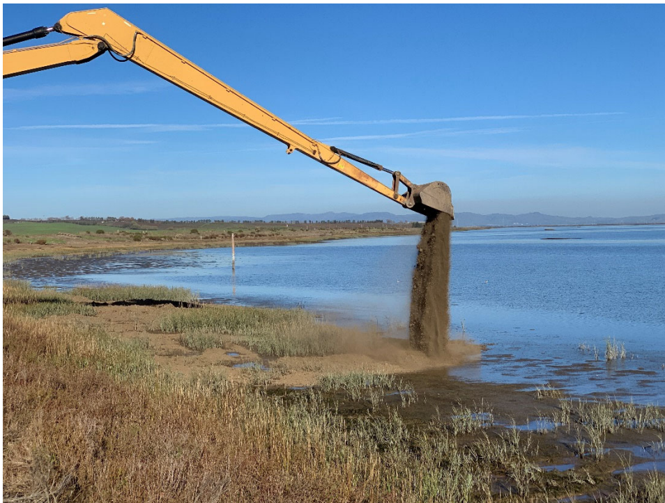
Photograph 9. Placement of Dry Aggregate Bay Mud Around Vegetation
