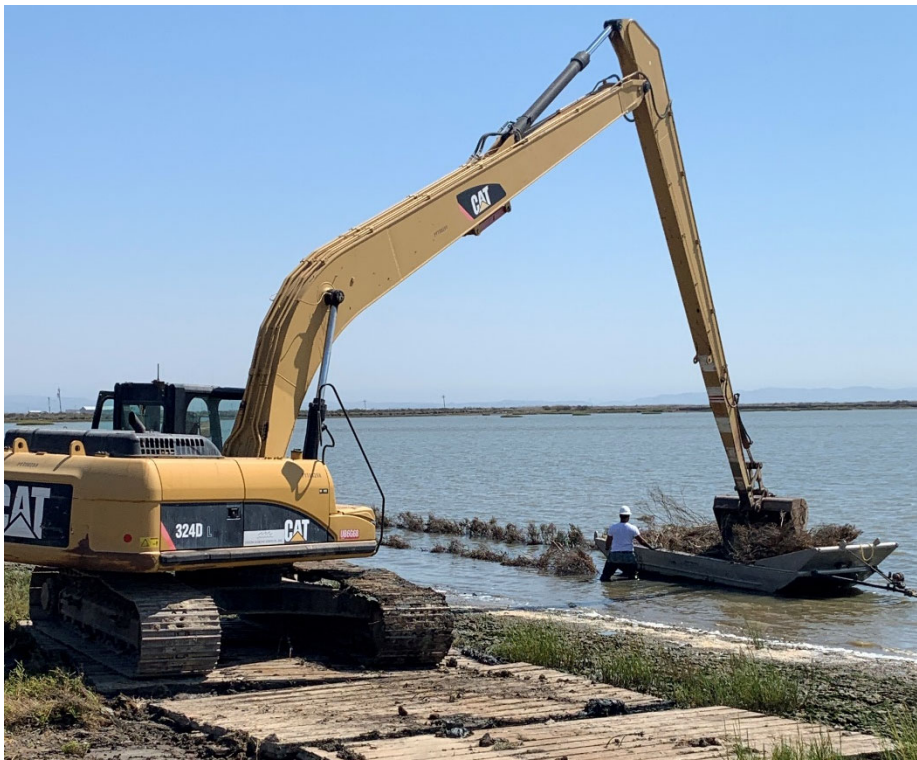
Photograph 8. Brush Fence Installation
