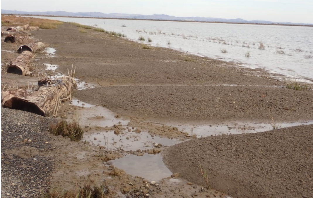
Photograph 10. Placement of Dry Aggregate Bay Mud Below Logs
