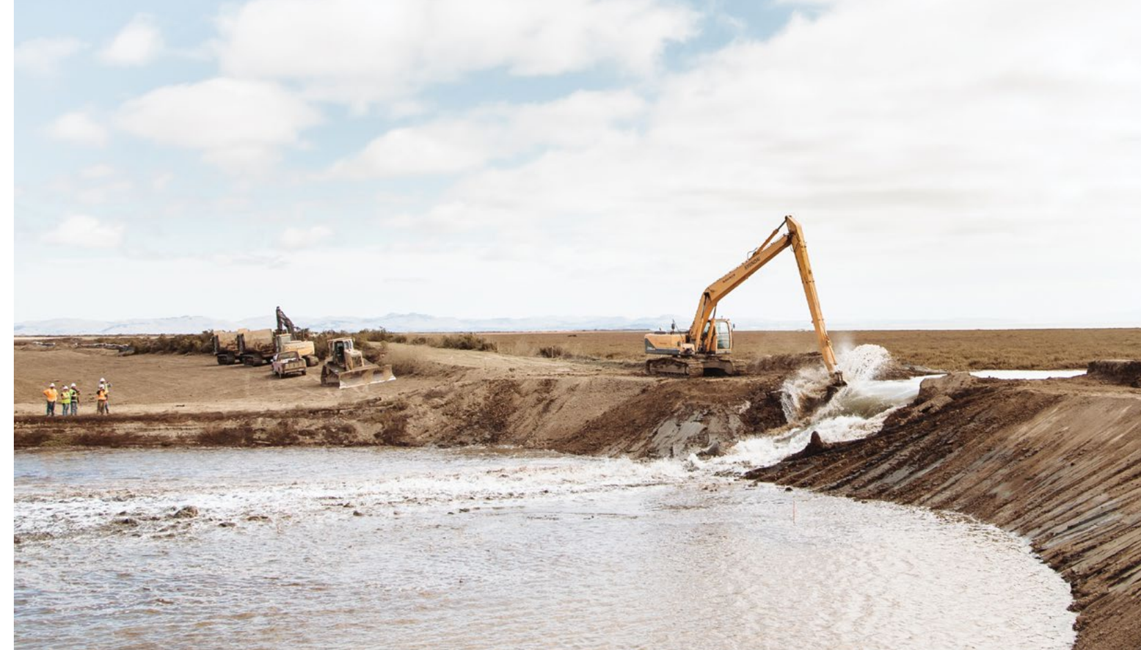
▲ An excavator breaches a levee at Sears Point, allowing tides back in for the first time in more than a century.
