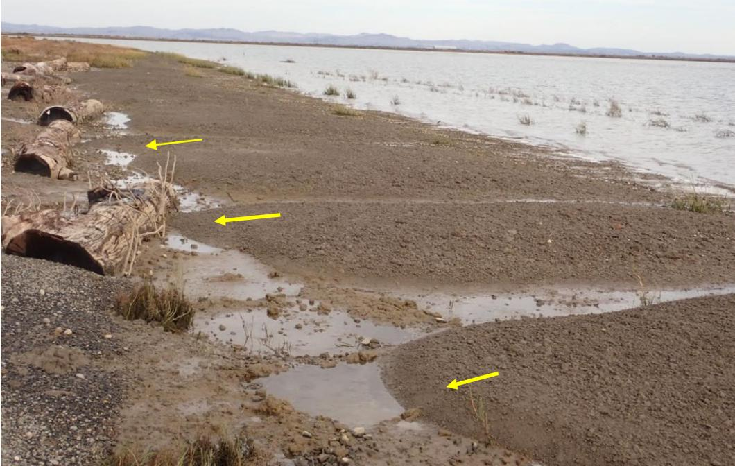
**Photograph 9. Rapid wave-reworking and drifting of aggregate bay mud mound deposits into swash bars during construction (2)**
