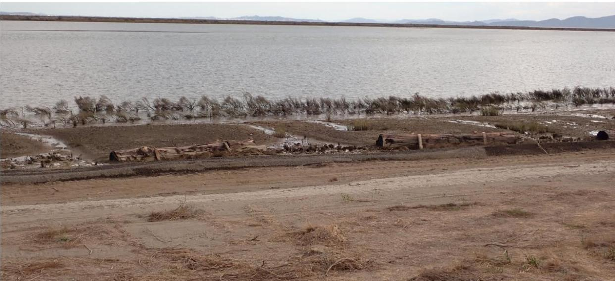
**Photograph 27. Cross-shore distribution of all dynamic, interacting “nature-based” shoreline stabilization elements in Cell 6 with completed construction**
