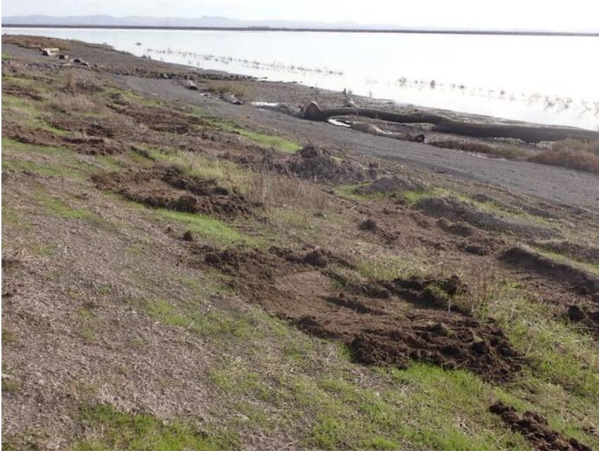
**Photograph 29. Staggered series of planted, buried large creeping wildrye sod mat fragments on levee slope above the high tide line**
