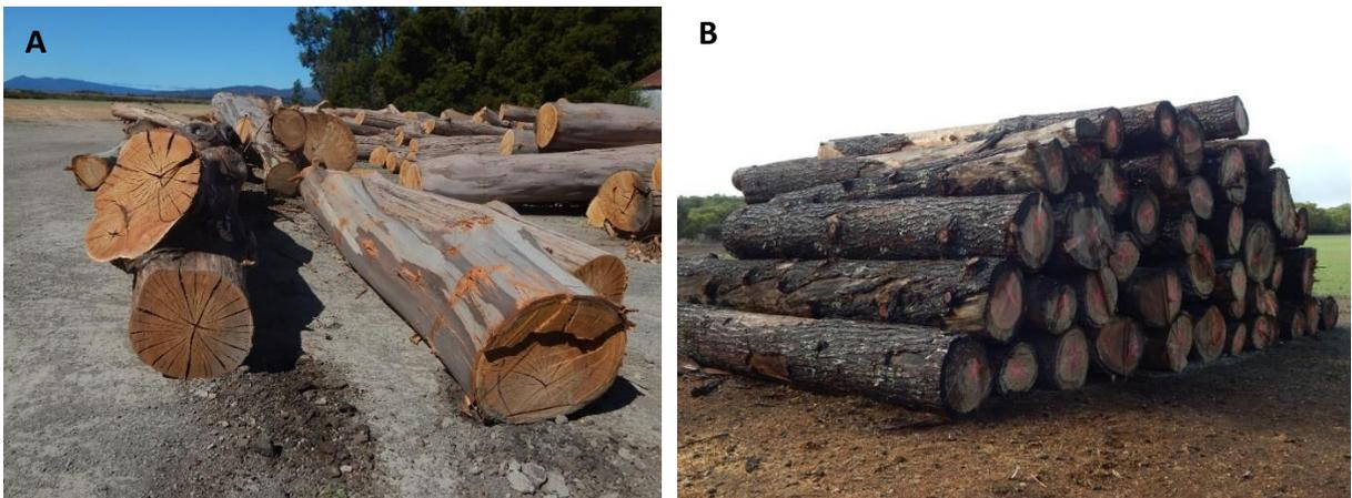
**Photograph 13. Raw logs stockpiled on-site for shoreline placement as artificial analogs of driftwood**
