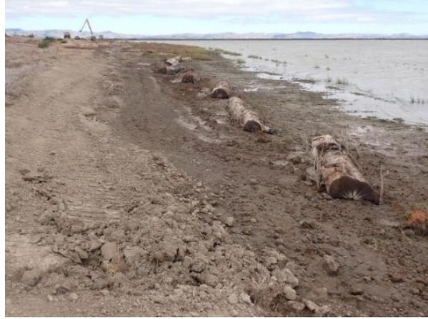
**Photograph 15. Series of installed embedded logs**
