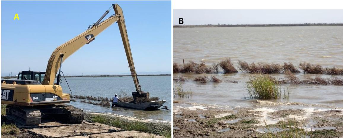
**Photograph 1. Brush fence installation on inner mudflat cordgrass transplant zones**
