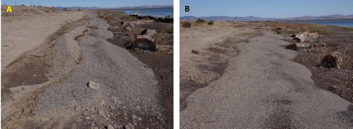
**Photograph 21. Near-complete wave-reworking of sacrificial gravel berms into swash bars**
