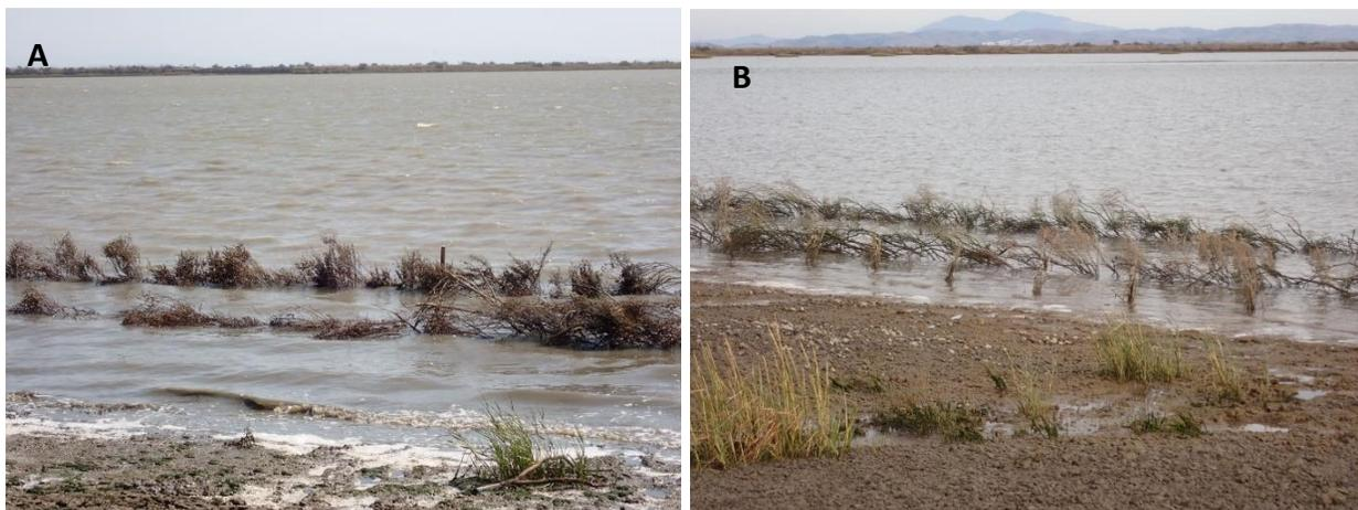
**Photograph 2. Brush fence early post-construction functions**
