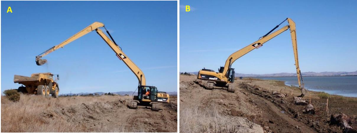
**Photograph 5. Placement of aggregate bay mud on eroded wave-cut levee bench**
