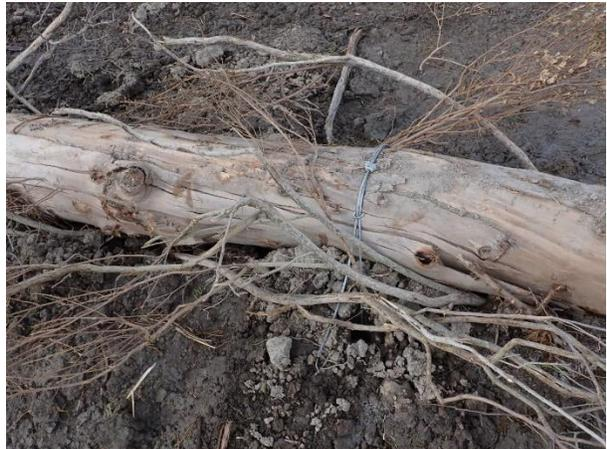
**Photograph 16. Cabled and anchored embedded eucalyptus logs**
