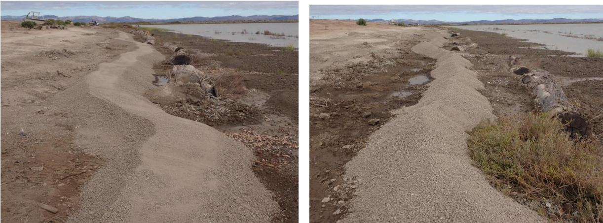
**Photograph 18. Freshly deposited, dry, unconsolidated sacrificial gravel berms**
