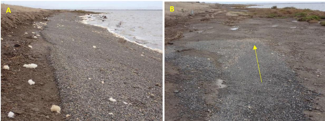
**Photograph 24. Evolution of gravel swash bars in late fall, weeks after gravel placement**
