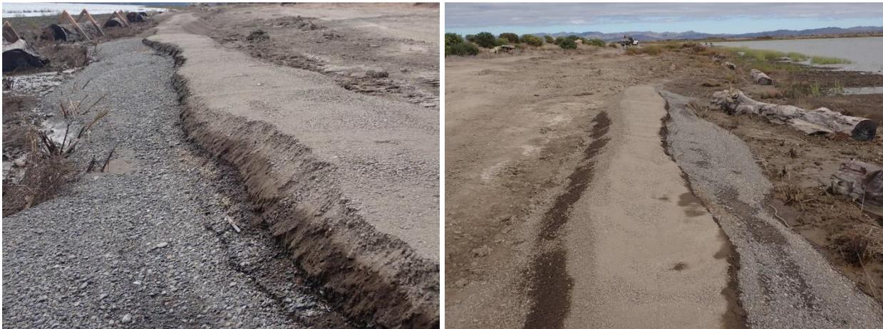
**Photograph 20. Initial partial wave-reworking of sacrificial gravel berms**
