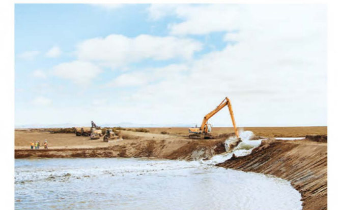
In October 2015, the old levee at the Dickson Ranch Unit was breached, returning the tides to 1,000 acres of former marshland.
