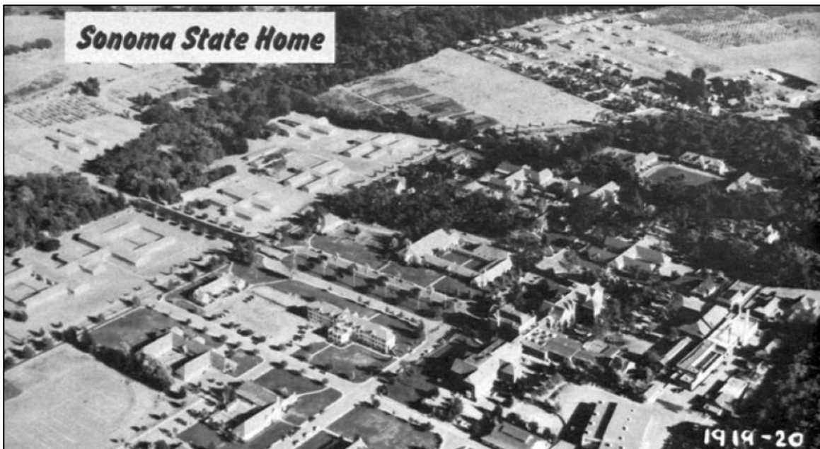
Aerial view of the facility from 1919-20. Photo from the Asylum Projects.
